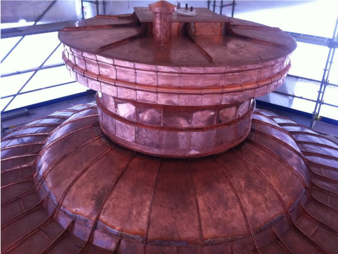
Finished copper work before railing installation.
