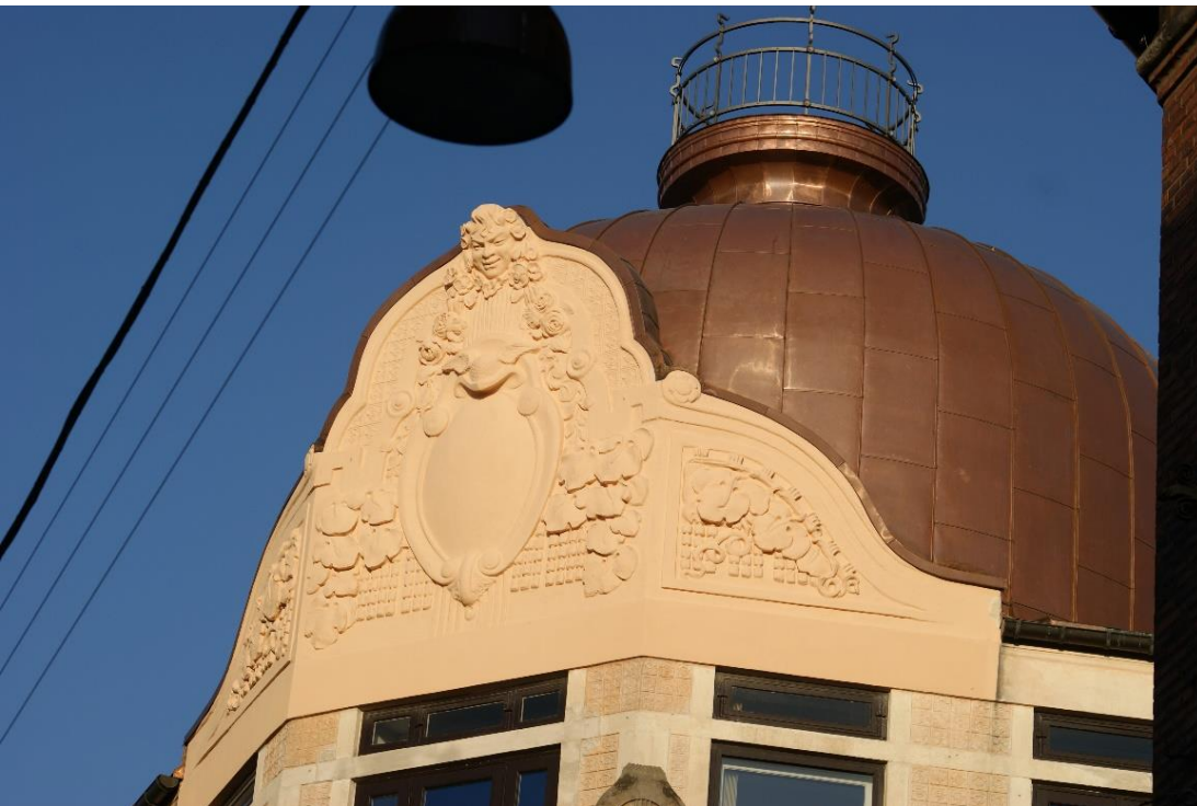
Finished copper work before railing installation.
