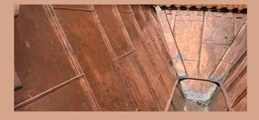
At Grundtvig's Church, the last copper vessels on each side of the nave have now been replaced. The copper vessels are not visible from below at street level.
