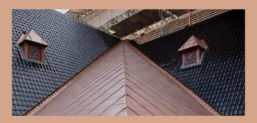
On the 4 areas of the roof where there is copper, the old green roof was installed and replaced. In addition, 16 copper rafters in the tiled roof were renovated, new ventilation hoods and vents, stern, gutters and downspouts were installed on the entire roof - all done by hand.
